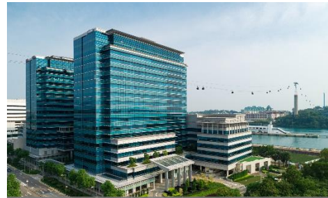
Keppel Bay Tower, Singapore
