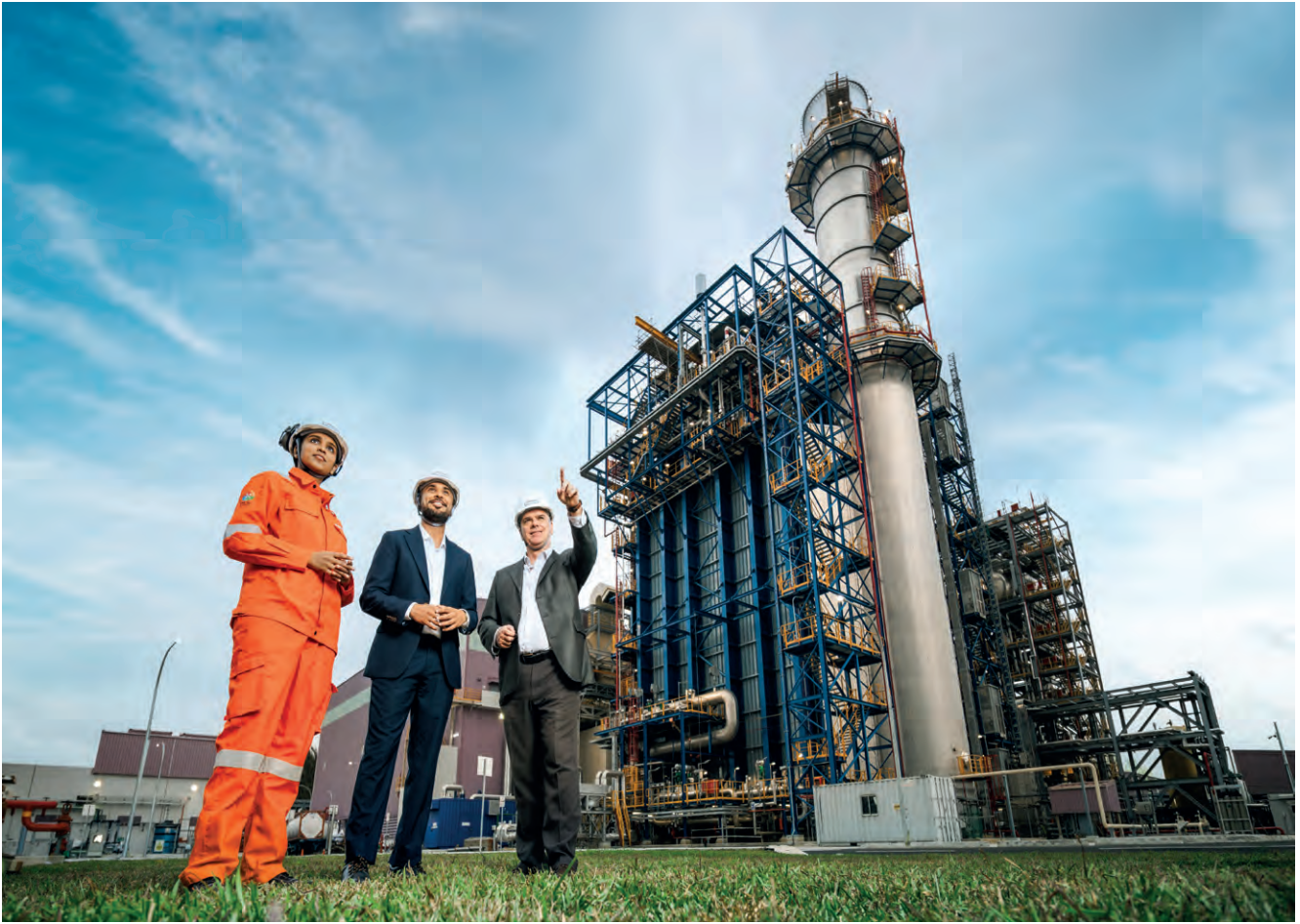
Keppel Sakra Cogen Plant, Singapore's most advanced and first hydrogen-compatible advanced combined cycle gas turbine power plant, is on track to achieve generation readiness in 1H 2026.
