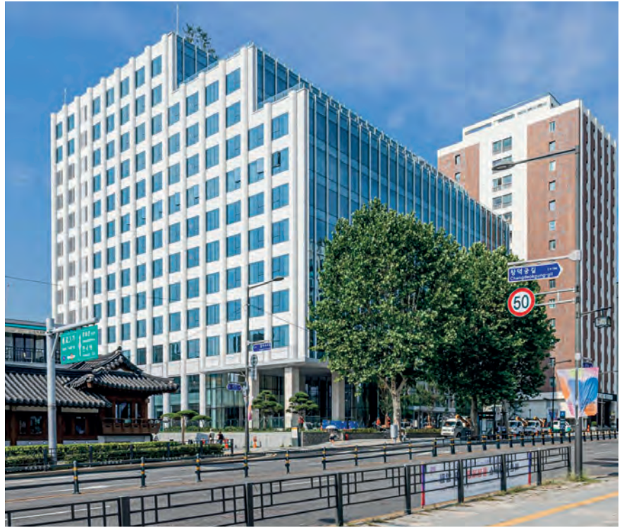
At the more than 40 year old INNO88 Tower in Seoul, Keppel incorporated various sustainability features such as high-performance building facades to improve the asset's operational efficiency and performance.
