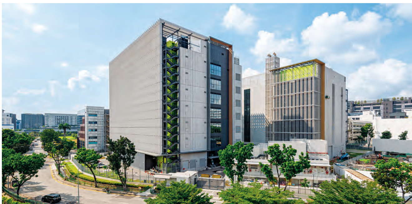
Keppel DC Singapore 8, an AI-ready hyperscale data centre situated within the Keppel Data Centre Campus, achieved the BCA Green Mark Platinum Award, the highest green accolade conferred by BCA for new data centre developments.
