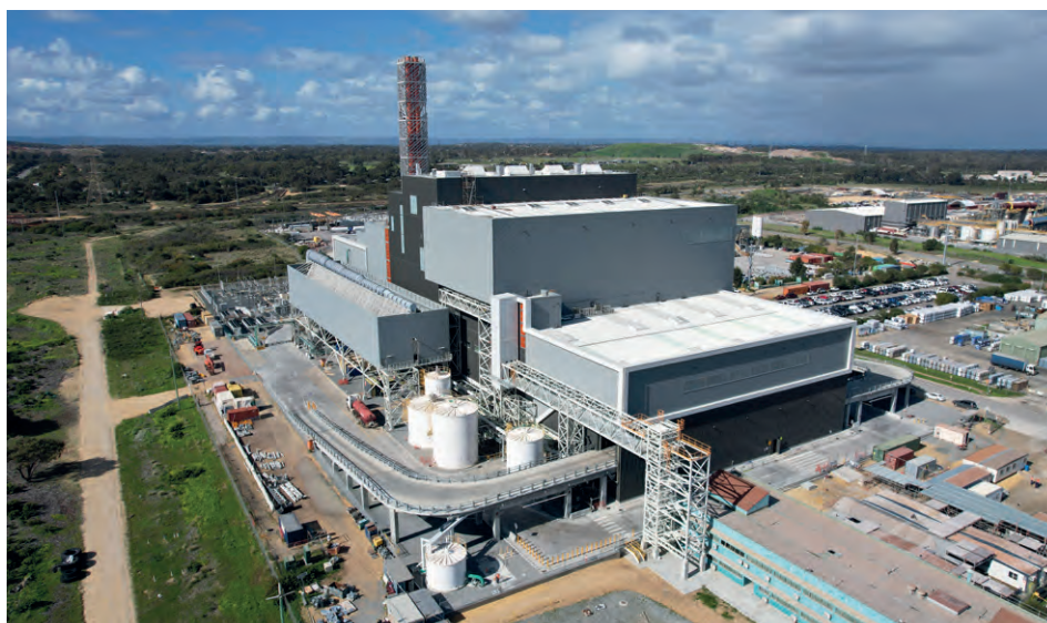
The Kwinana Energy Recovery Facility in Perth, Western Australia, features Keppel's waste-to-energy technology.
