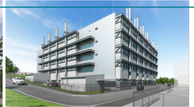
Western Tokyo Data Centre
