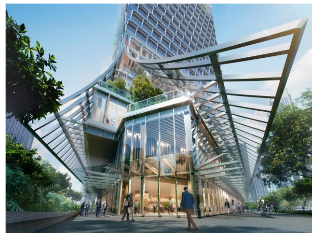
Keppel South Central is a BCA Green Mark Platinum Super Low Energy certified building
