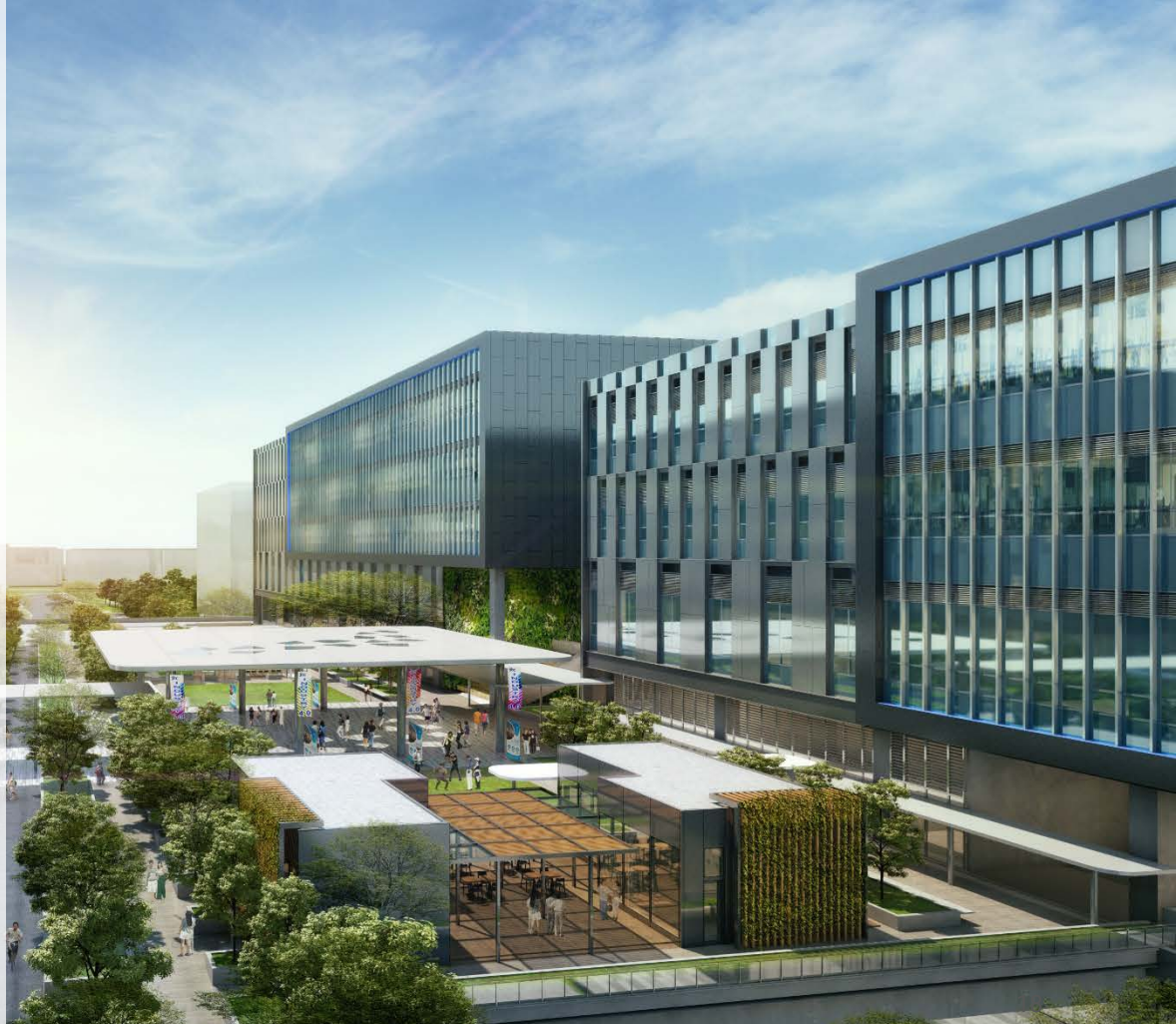
Artist's impression of Bulim district cooling system plant in Jurong Innovation District, Singapore
