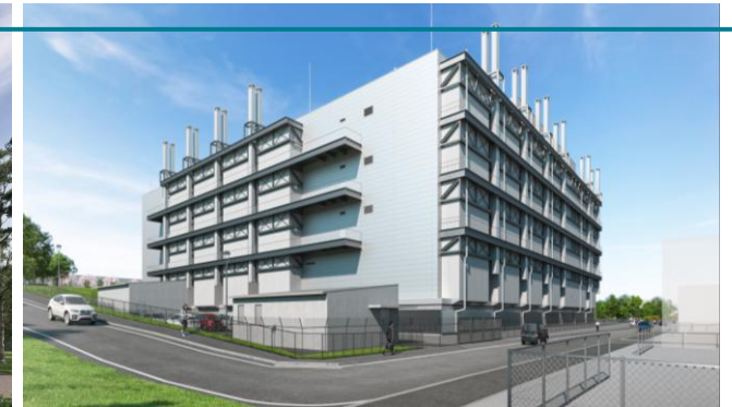
Western Tokyo Data Centre
