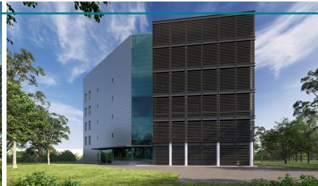
Taiwan Data Centre Campus
