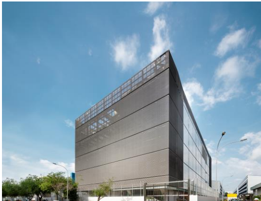
Keppel DC Singapore 4, Singapore
