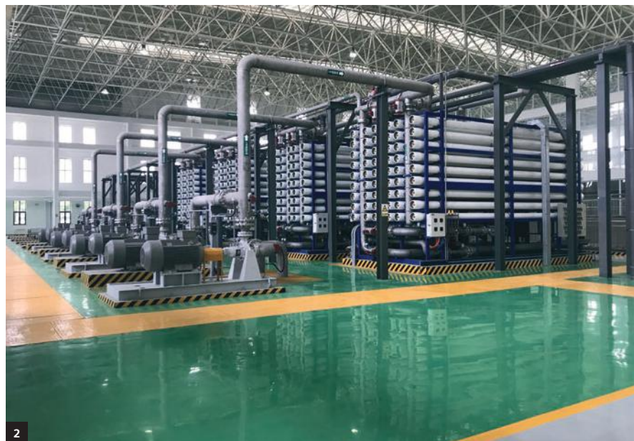
2. The Sino-Singapore Tianjin Eco-City Water Reclamation Centre treats wastewater effluent to produce recycled water that meets China’s most stringent standards.
