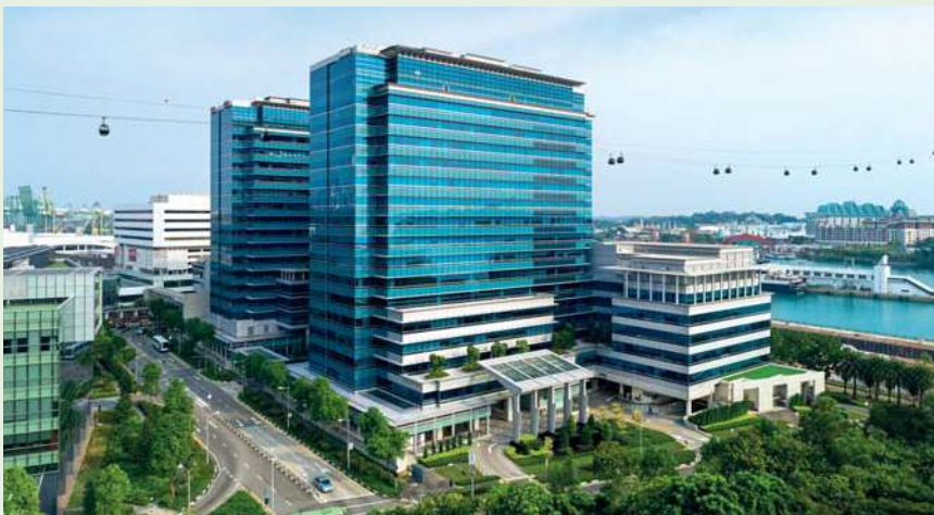
In January 2020, Keppel Bay Tower became Singapore's first commercial development to be fully powered by renewable energy.
