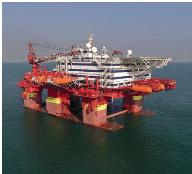
Keppel FELS delivered Floatel Triumph, a high-specification accommodation semi, safely and on time.
