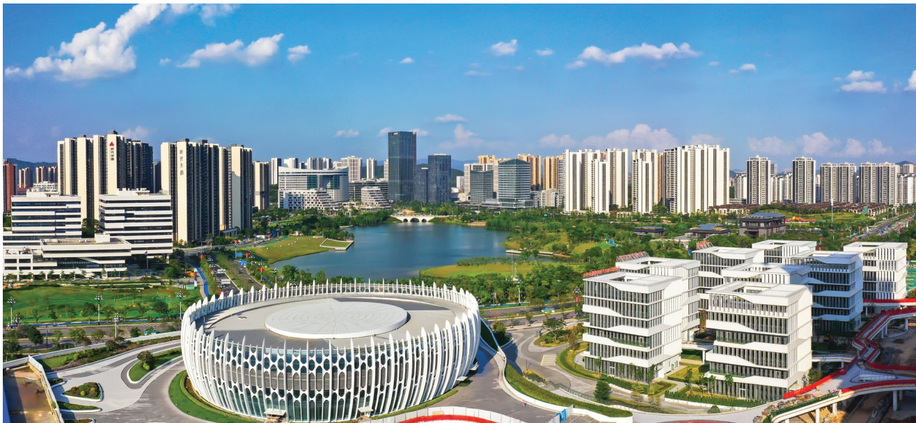
Keppel and GKC JV Co are currently planning the roll-out of EaaS at sites in CSGKC, such as the China-Singapore Smart Park (CSSP), located in the Start-Up Area.
