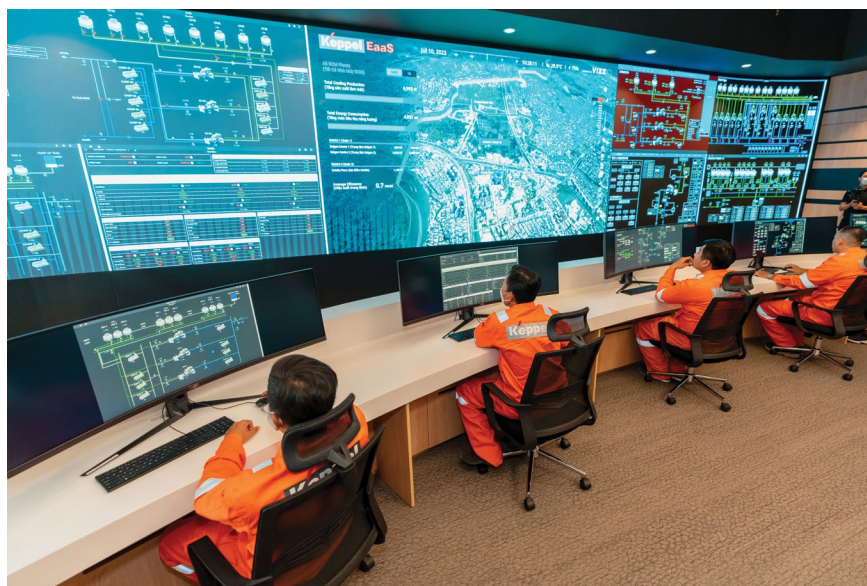
Keppel's Operations Nerve Centre, housed in Thu Duc City, will be able to remotely monitor and optimise all of its energy assets in Vietnam in real time, leveraging digital technology, artificial intelligence and machine learning.
