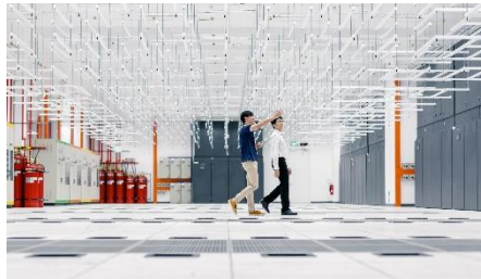
Data hall fit out
