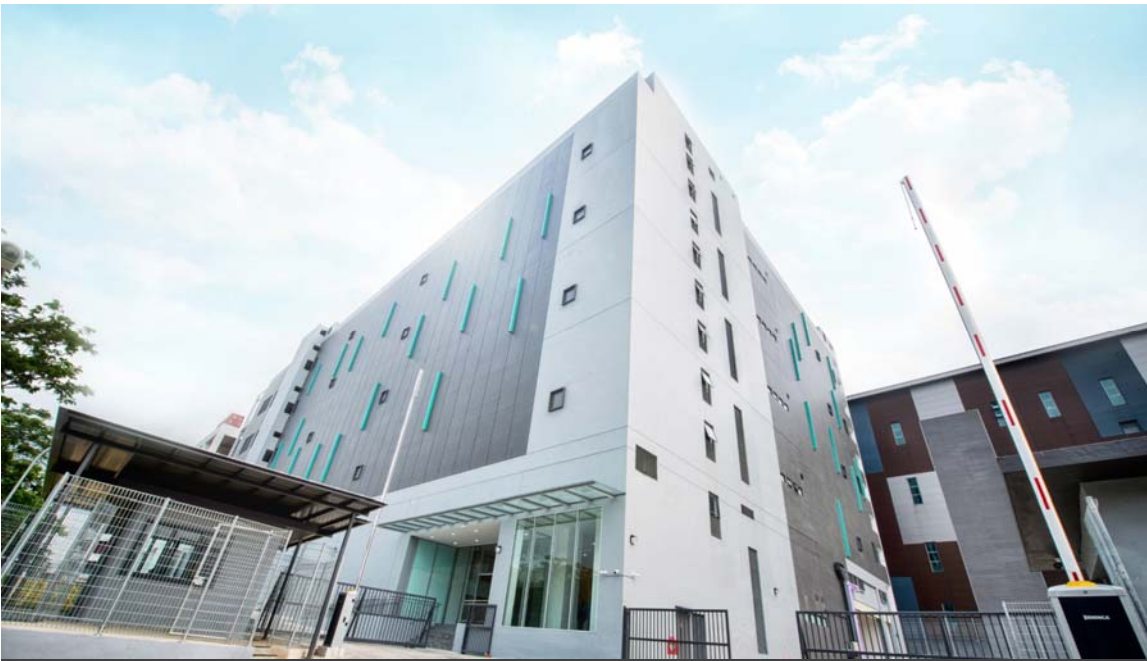
Keppel DC REIT completed acquisition of Keppel DC Singapore 5
