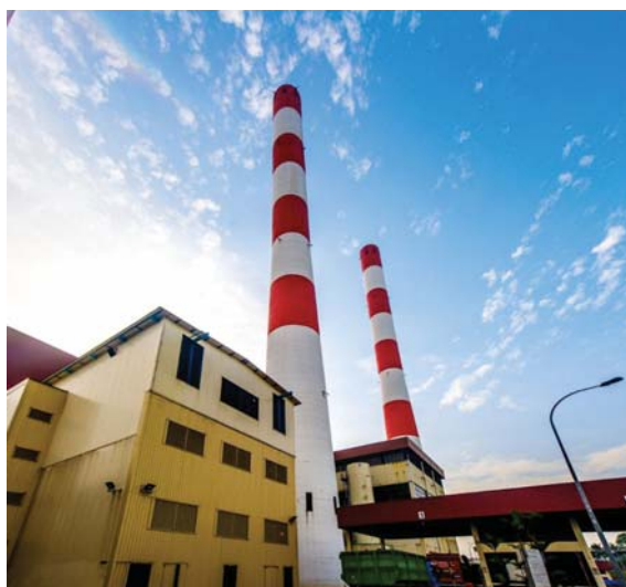
Senoko WTE plant, Singapore
