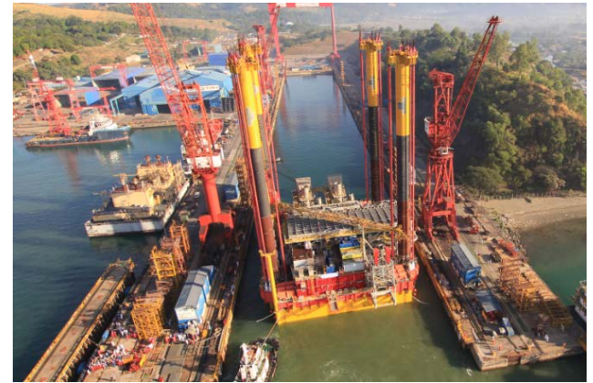
Shell's Depletion Compression Platform
