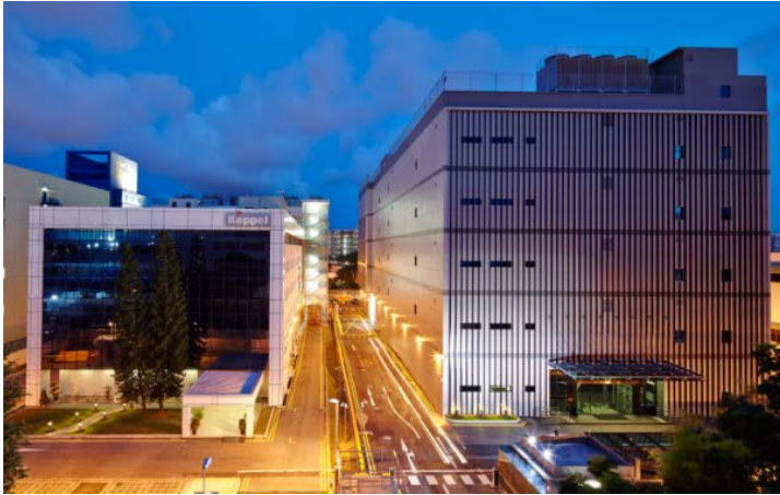
Keppel Datahub 2 (right)
