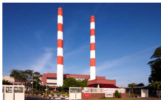
Senoko WTE Plant, Singapore
