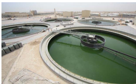
Doha North Sewage Treatment Works, Qatar
