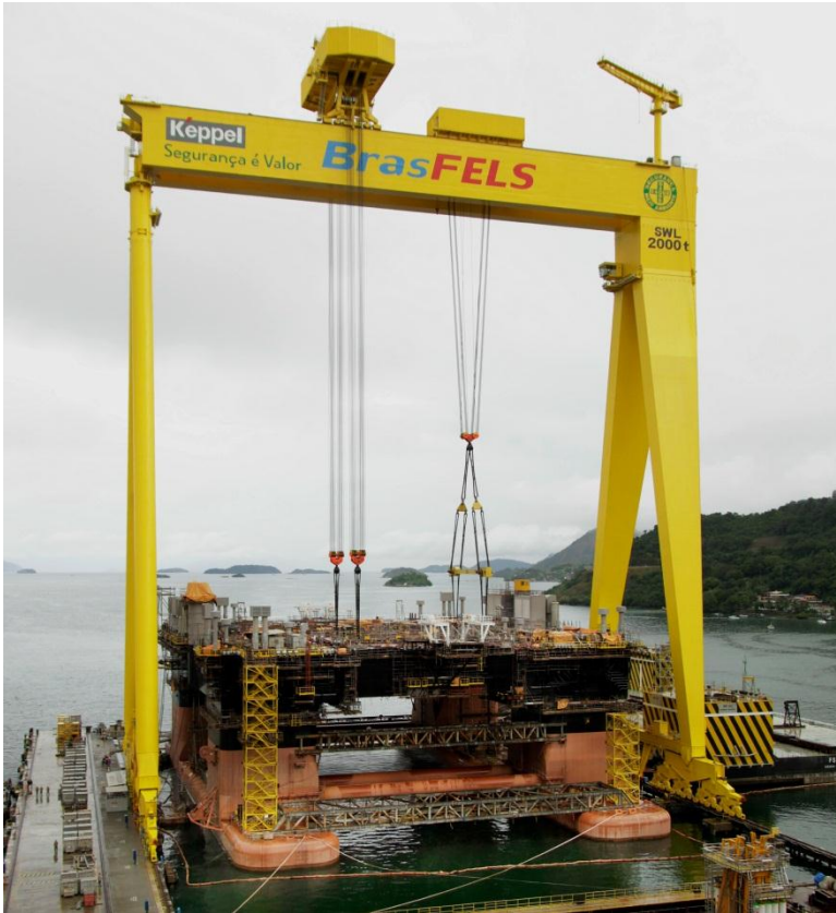
First DSS™ 38E semi under construction at Keppel FELS Brasil's yard in Angra dos Reis
