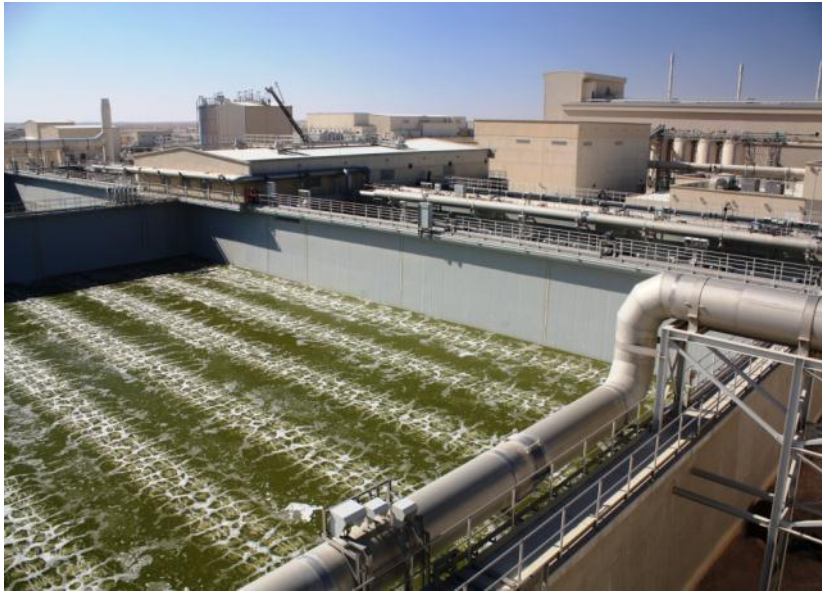
Doha North Sewage Treatment Works, Qatar
