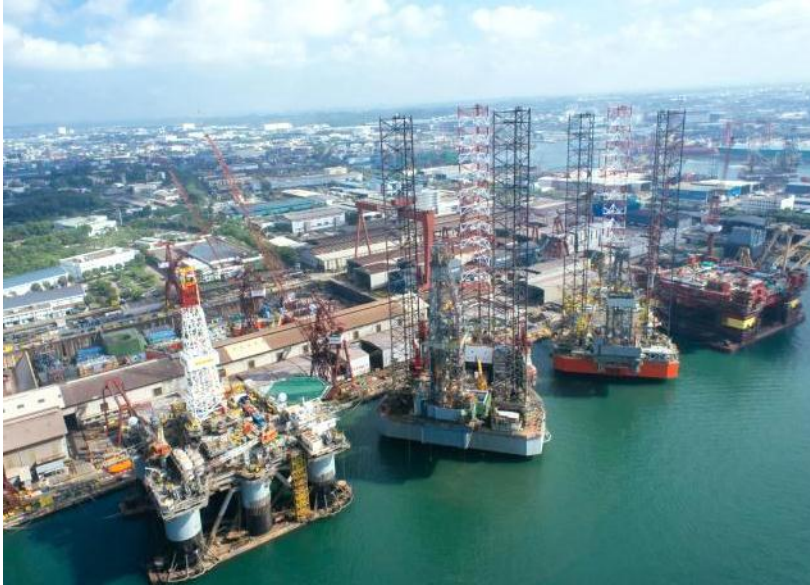
Keppel FELS, Singapore
