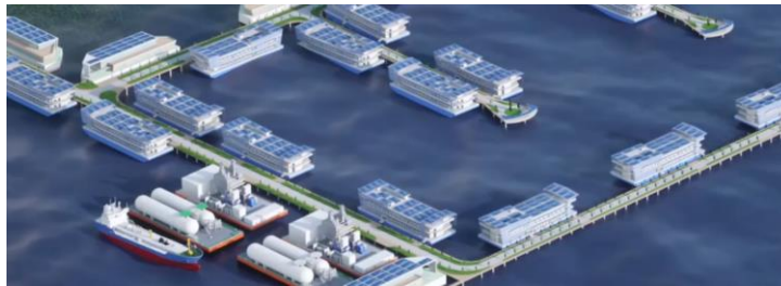
Floating data centre park
