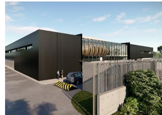
IndoKeppel Data Centre 1, Indonesia
