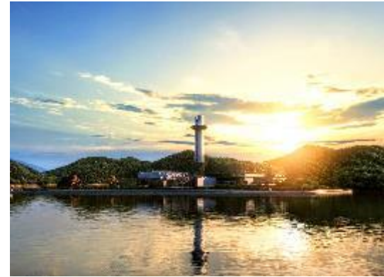
Hong Kong Integrated Waste Management Facility (HKIWMF)
