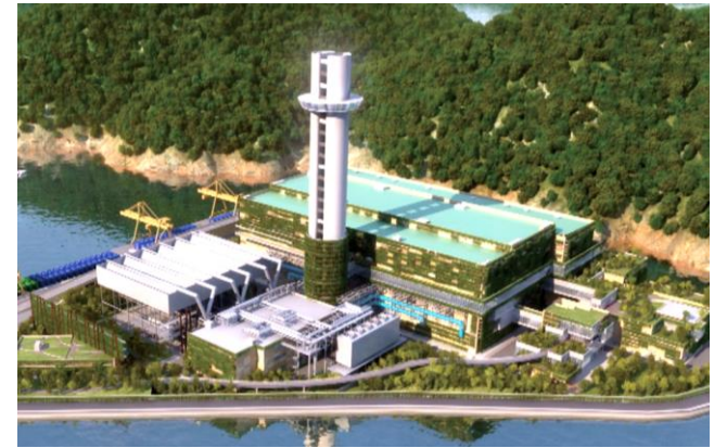
Integrated Waste Management Facility, Hong Kong
