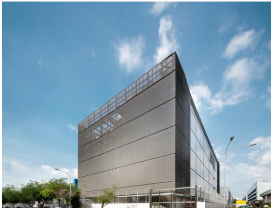
Keppel DC Singapore 4, Singapore
