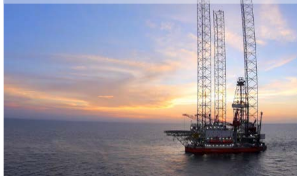
Cantarell I and II operating in Mexico
