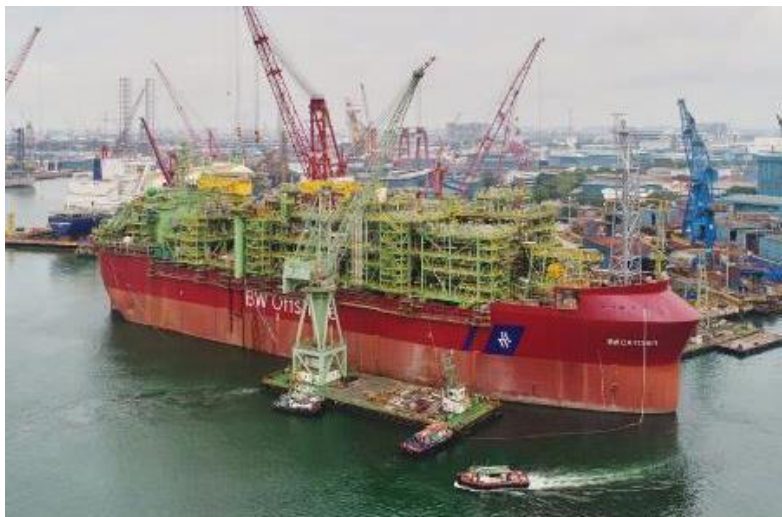
BW Catcher - FPSO Hull and marine systems completion and topsides integration
