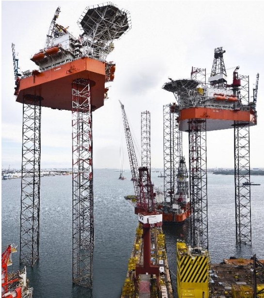
KFELS B Class jackups, CANTARELL I & II
