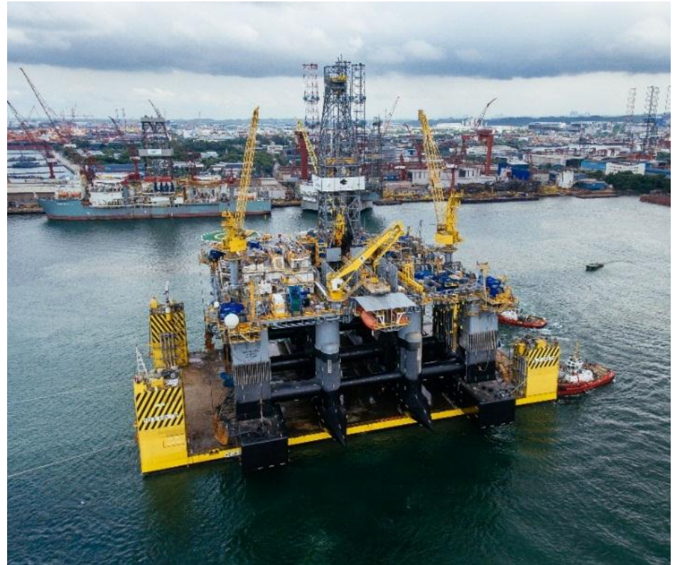
Refurbishment of semi, Ocean Apex
