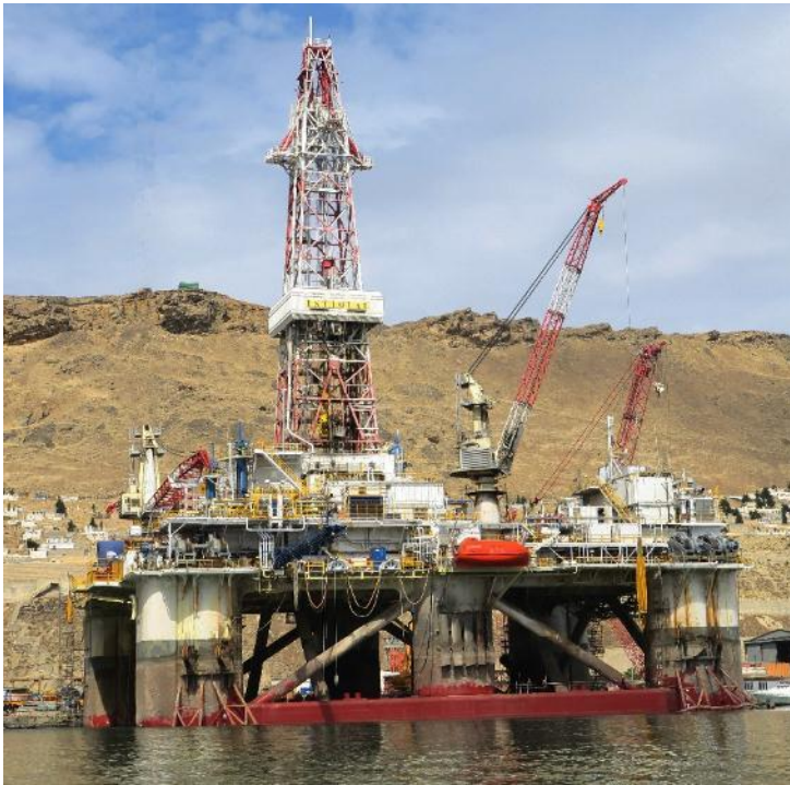
Upgrade of semi drilling rig, Istiglal
