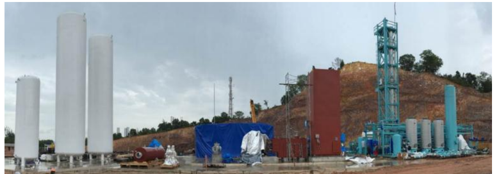
The land-based PreNEx LNG plant for PT NAT Gas has a liquefaction capacity of 50 tons/day.
