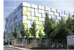
maincubes Data Centre*, Germany
