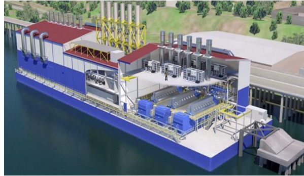
Single/Dual Fuel Floating Power Barge
