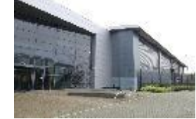
Data centre in Cardiff*
