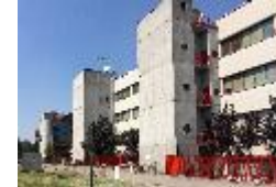
Data centre in Milan*
