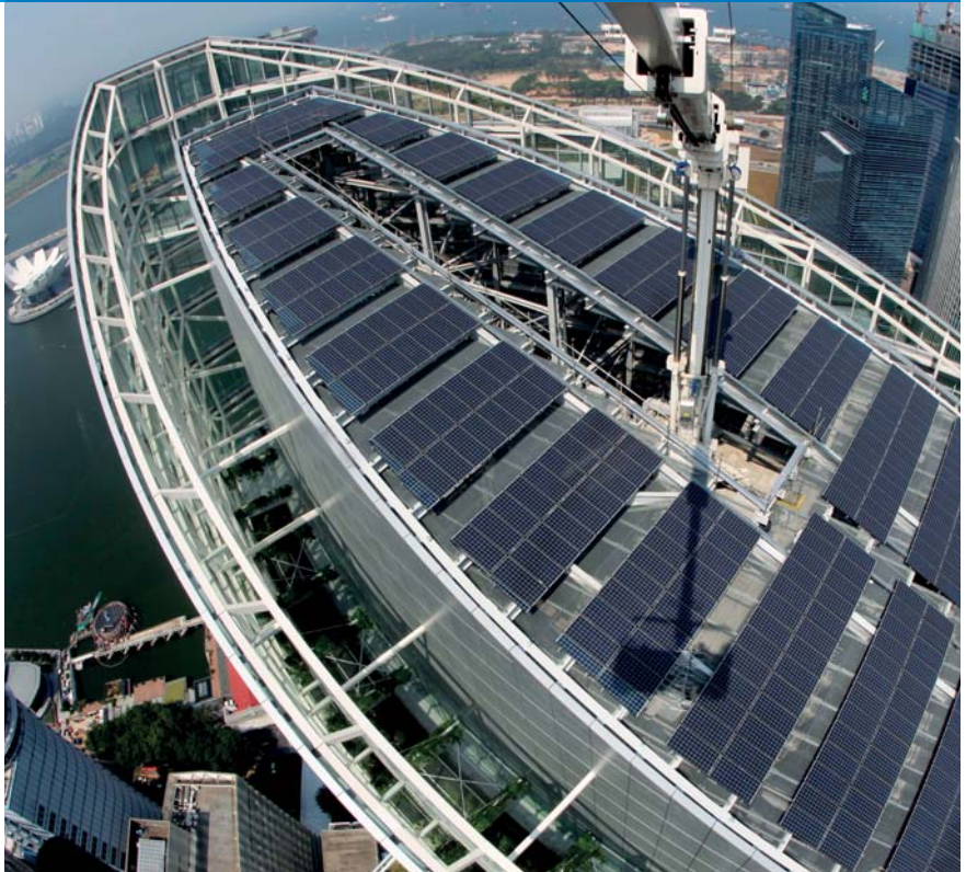
Ocean Financial Centre is retrofitted with solar panels that can generate 86 megawatt hours worth of clean energy in a year.
