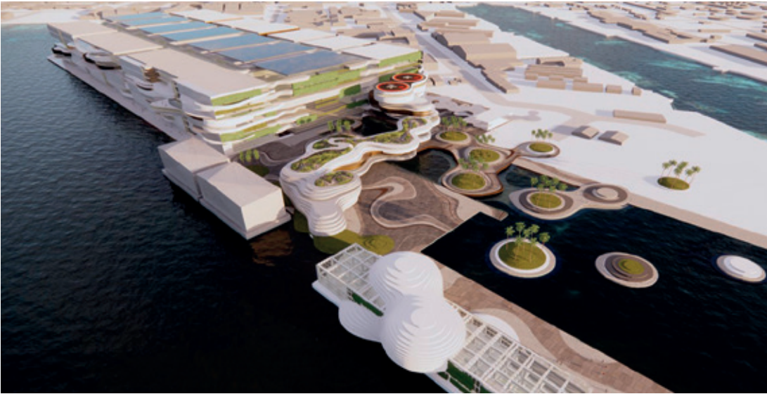
The proposed DataPark+ is a 1 GW nearshore sustainable data centre campus that is envisioned to be powered by hydrogen and solar energy, and can save nearly 21 billion litres of water annually through the use of seawater for cooling.
