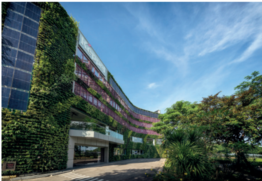
KI@Changi, Singapore's first Green Mark Platinum Positive Energy building under the new Green Mark scheme.
