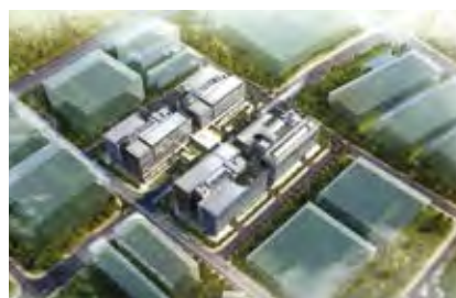
Keppel DHCS will build, own and operate a DCS plant in Bulim Phase 1 of Singapore's Jurong Innovation District.
