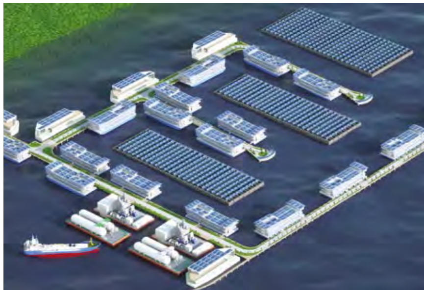
As part of Vision 2030's focus on sustainability, Keppel is exploring the development of floating data centres, which are more energy efficient than traditional land-based ones.
