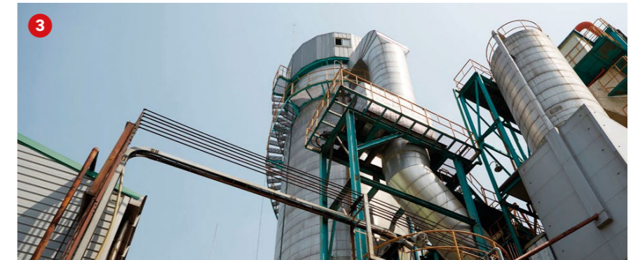
Expanding capabilities in environmental infrastructure.
