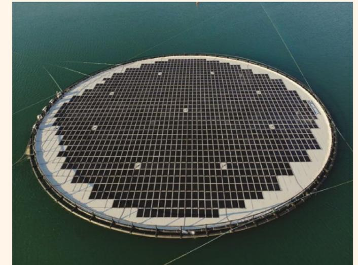
Keppel Infrastructure was awarded a grant from the Energy Market Authority (EMA) and JTC to pilot Singapore's first membrane-based nearshore floating solar photovoltaic (PV) system at Jurong Island. The pilot PV system consists of three circular platforms, which will have an installed capacity of 1.5 MWp.
