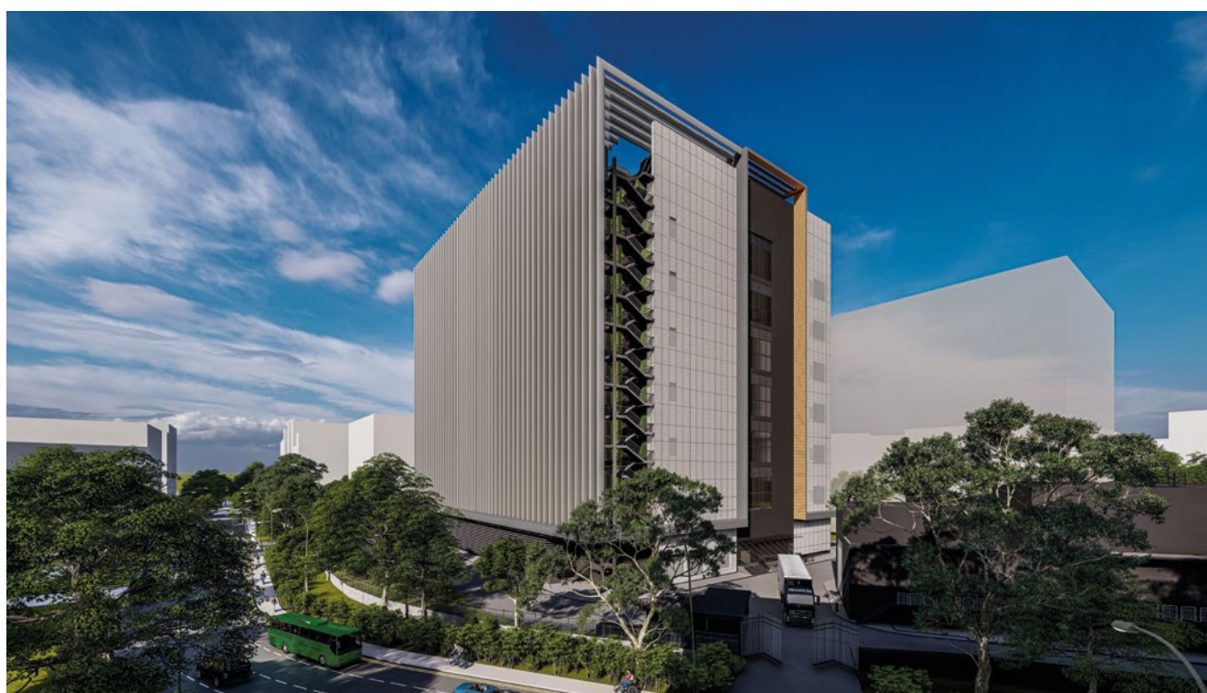
KDC SGP 7 in Genting Lane has achieved the BCA Green Mark Platinum Award, based on the Green Mark for New Data Centres. This is the highest green accolade conferred by Singapore's BCA specifically for new data centre developments. The data centre incorporates green features such as energy-efficient equipment and advanced technologies to improve performance of the chiller plant and data hall cooling systems, as well as reduce water consumption.
