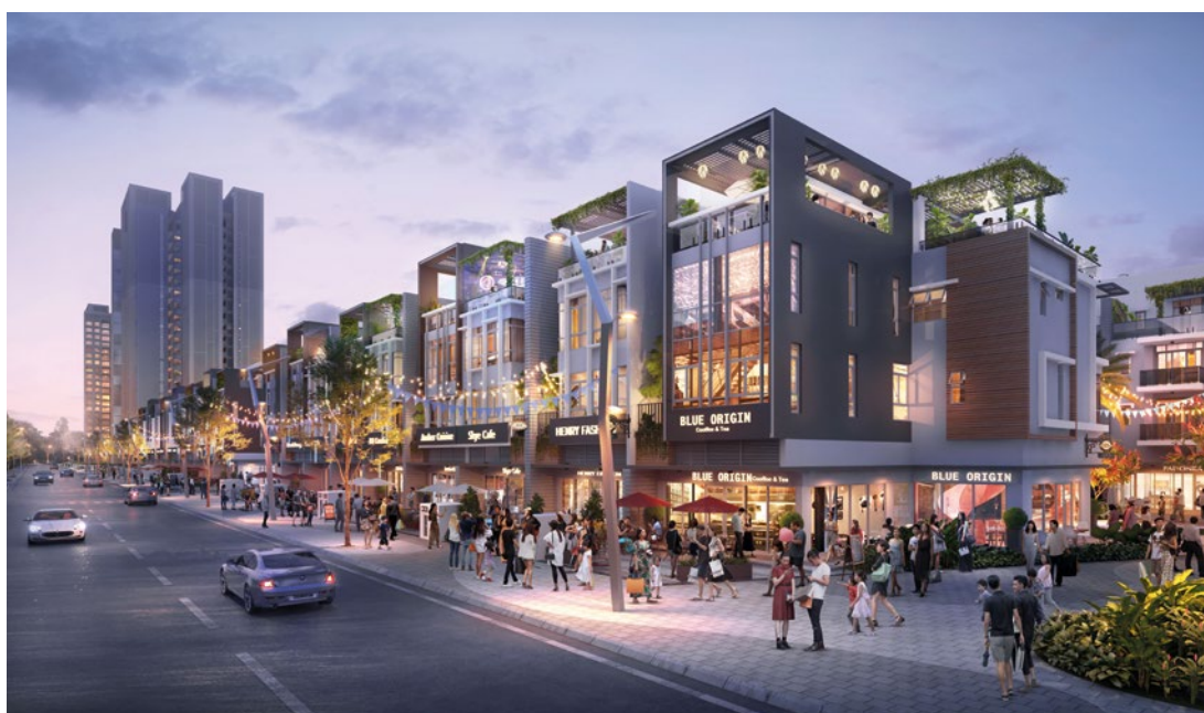
Keppel Land has built a strong and diverse track record in Vietnam, winning several industry-leading awards and drawing good buyer demand for its developments. (In picture: Celesta Avenue in Ho Chi Minh City, was named the Best Housing Development at PropertyGuru Vietnam Property Awards.)
