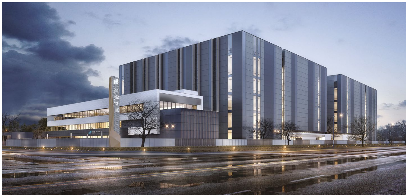
KDC Fund II entered a strategic partnership with Heying, a wholly-owned subsidiary of Tianjin Zhengxin Group, to jointly develop Huailai Data Centre, a greenfield data centre in Greater Beijing.
